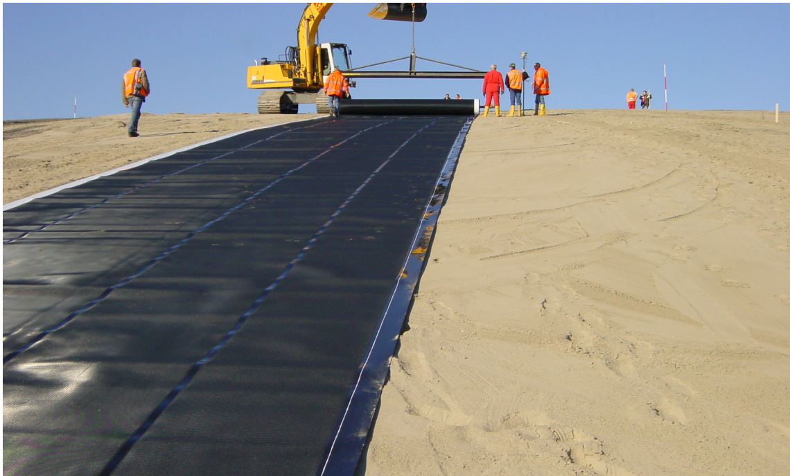
Figure 3. Construction of an impermeable hdpe top liner.
