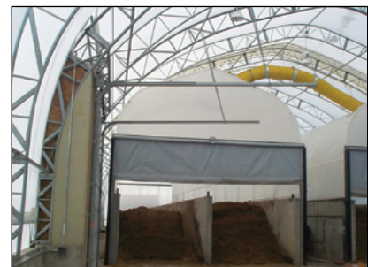
Photo 5-25: Channel composting system © Scott Gamble
