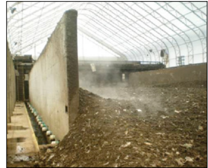
Photo 5-26: Agitated bed system viewed from discharge end of bay © CH2M HILL
