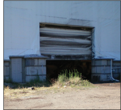
Photo 9-7: Leaving doors open impairs the ability of a building's ventilation systems to contain odours © CH2M HILL
