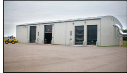
Photo 10-3: Engineered steel frame receiving building © CH2M HILL
