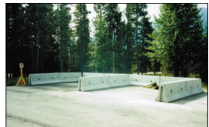
Photo 5-6: Small bunker composting system © Scott Gamble
