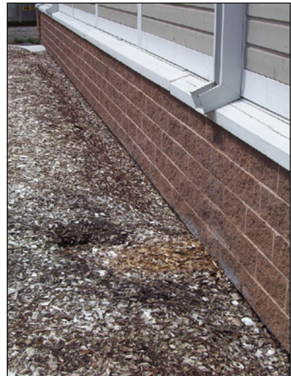
Photo 10-11: Water from roof drains should be directed around operating areas to minimize the quantity of contaminated surface water that has to be collected and treated © Scott Gamble
