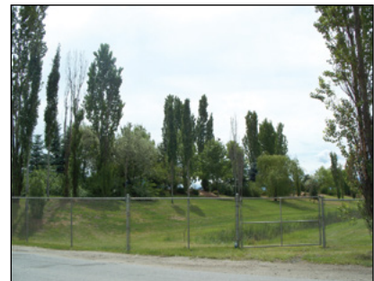
Photo 15-6: Soil berms and trees help reduce noise impacts, as well as improve visual appearances © CH2M HILL
