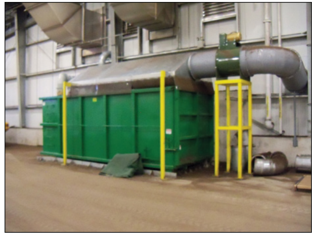
Photo 10-7: Enclosed roll-off containers can be used to contain litter and residuals from preprocessing and screening operations © CH2M HILL
