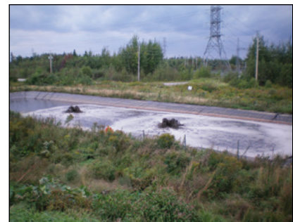
Photo 10-9: Contaminated stormwater is commonly collected in retention ponds and is reused in the treatment process © CH2M HILL
