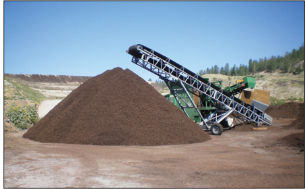
Photo 11-16: Stacking conveyors allow for the creation of large stockpiles with a small footprint © CH2M HILL
