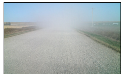
Photo 8-1: Unsurfaced roads can lead to significant dust impacts on neighbours © CH2M HILL
