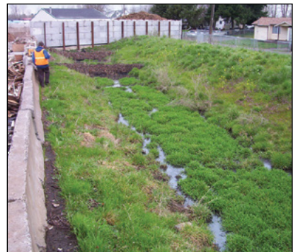
Photo 10-10: Filter berms and bioswales can be a cost-effective way to remove sediments from uncontaminated stormwater © Scott Gamble
