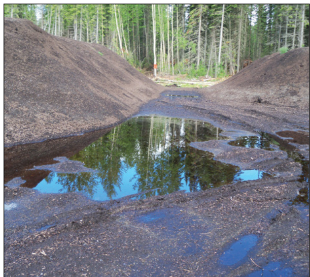
Photo 10-6: Water ponding in a compost facility's product storage area can affect access and lead to odours © CH2M HILL
