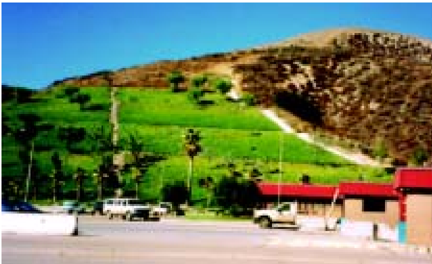
When the waste reaches a predetermined height, it is covered and planted with vegetation. The vegetation stabilizes the soil and gives the completed landfill a pleasant appearance.
