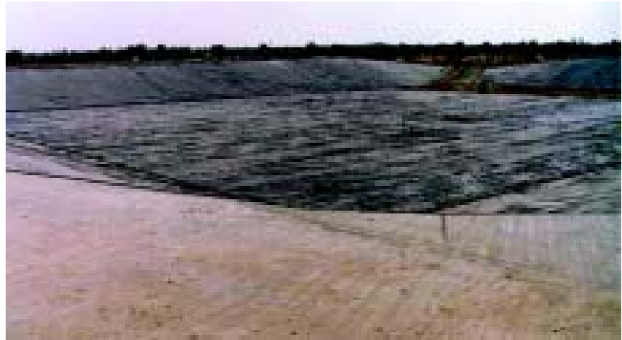
This landfill cell has been lined with an impermeable plastic liner so that underground water will not be polluted when solid wastes are placed in the cell.
