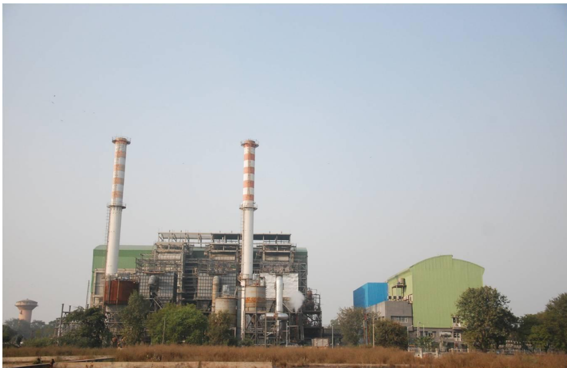
Fig.9. Jindal Incineration Plant, Okhla, New Delhi
